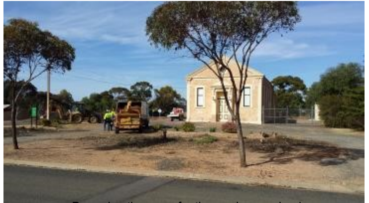
Preparing the area for the garden overhaul
