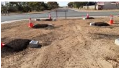
Holes and plaques ready to go
