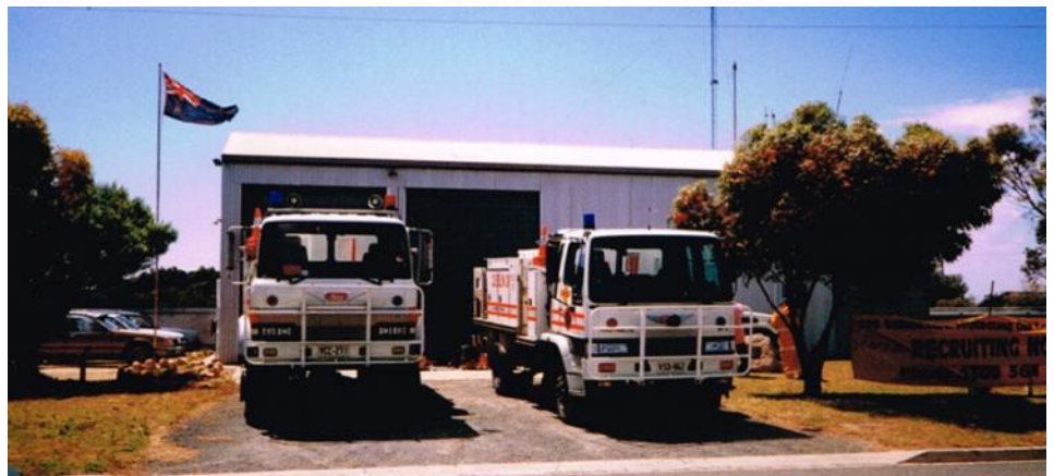
2001 SA CFS Dublin Station 6 First Street Dublin
